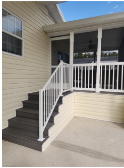
Staircase to front screen in porch
